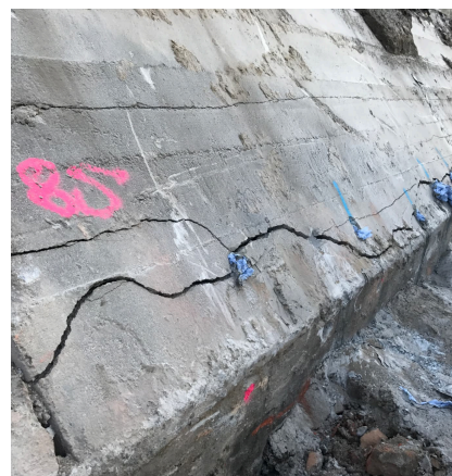
Concrete wall torn along the row of holes in a controlled way
