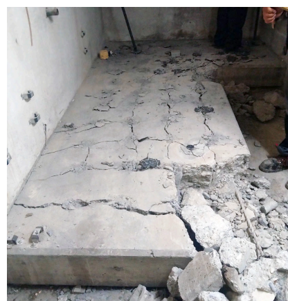
Concrete foundation demolished indoors
