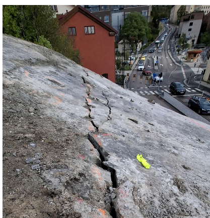
Rock removal above a busy road
