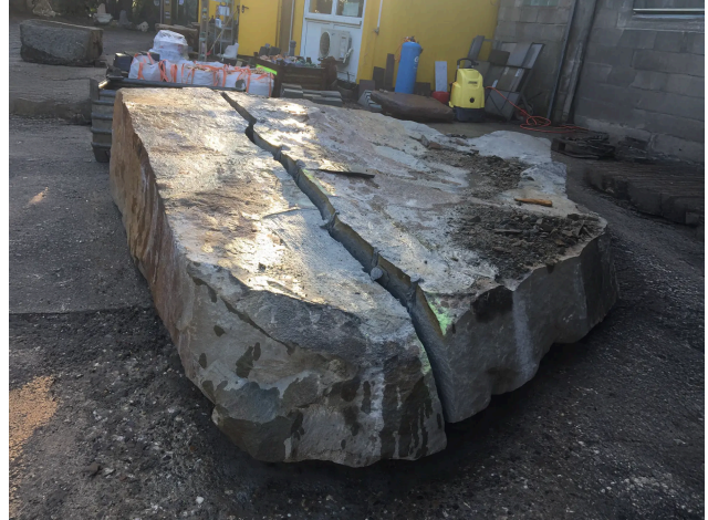
Boulder split without vibrations – no noise, no blasting.
