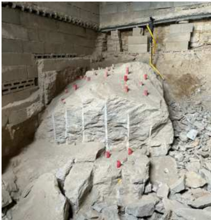
Rock breaking in cellar instead of chiselling
