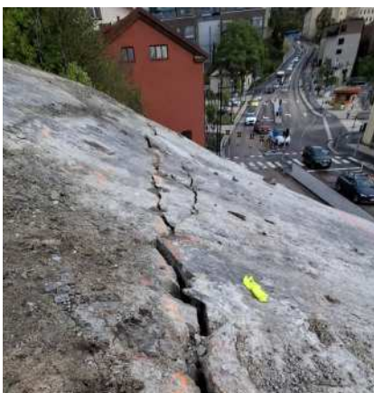
Rock removal above a busy road
