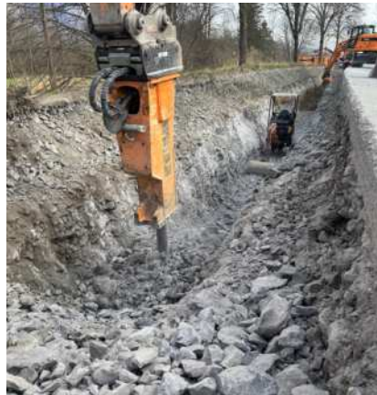
Trench excavation in rock – material loosened in advance
