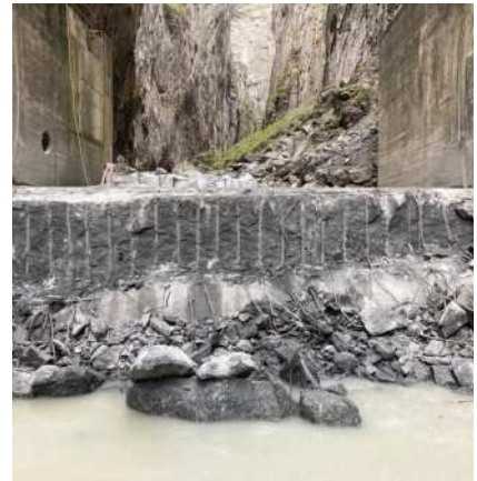
Dismantling of a concrete barrier in a gorge
