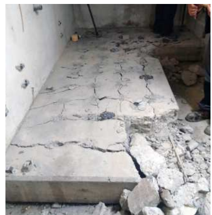
Concrete foundation demolished indoors
